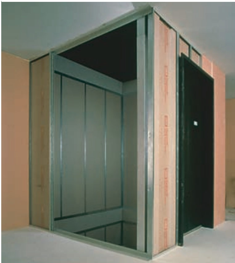
A TYPICAL SHAFTWALL SYSTEM DURING CONSTRUCTION FOR A LIFT APPLICATION
