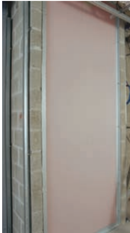
FIRST LAYER OF GYROCK FYRCEK AND PERIMETER FRAMING FIXED
