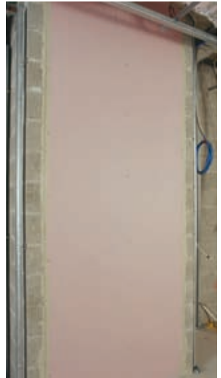
GYPROCK LAMINATED SERVICE SYSTEM AFTER COMPLETION
