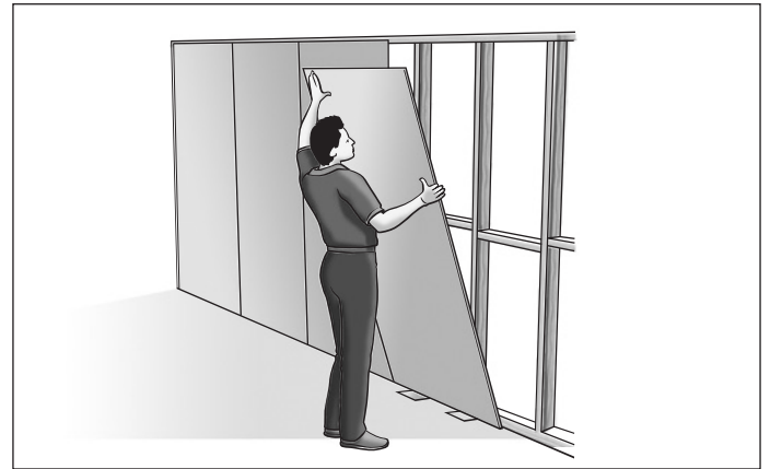
FIGURE 4 SHEET INSTALLATION
