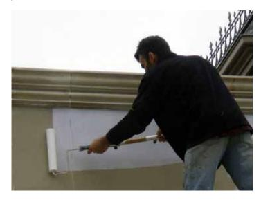
Because of the heavier texture provided by roll-on coatings, these products are ideal for application over irregular or roughly finished surfaces. They also provide for excellent hiding of shrinkage cracks with just one coat. Typical coverage is 16-18m² per pail for fine texture and 8-10m² per pail for heavy texture. Of course coverage rates vary with the surface condition.
