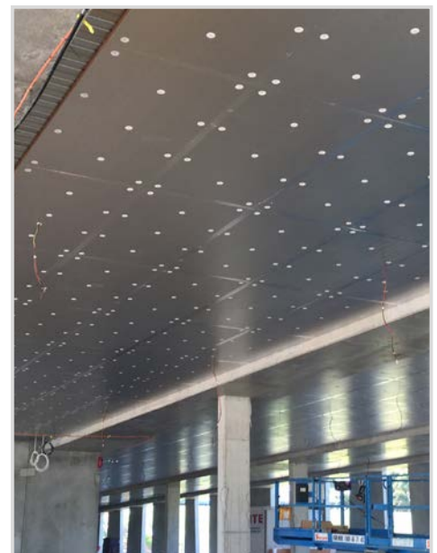
Press trigger of tool to fasten nail into base material - fixing complete.
