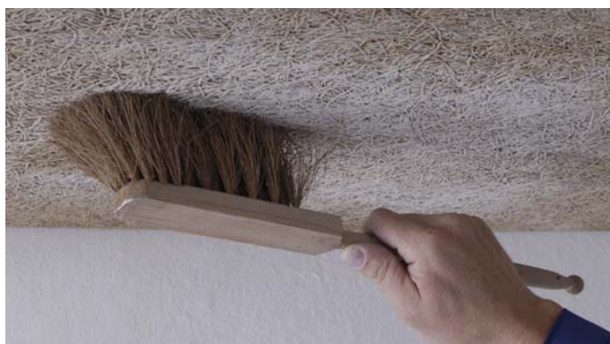
Brushing – Efflorescence, dust, etc. can be removed with a soft brush. Set loose fibres with a commercial grade acrylic primer.
