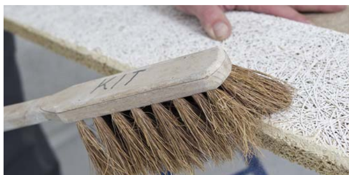
Remove any dust with a soft brush.
