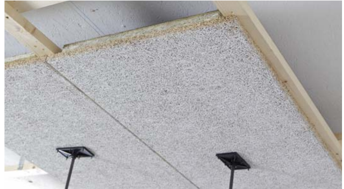
Installing the first row of panels: always start installing from the centre of the room, which has been pre-marked. Exactly align the panels in longitudinal and transverse direction.
