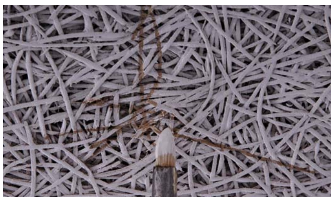
Chipped fibre – Cover chipped fibre with a fine brush or a spray gun using the supplied paint or an equivalent.
