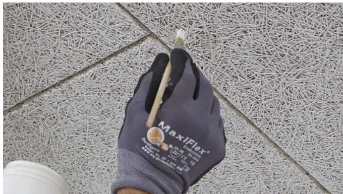
Painting over the screw heads – Use a fine brush to cover unpainted screw heads with the colour of the panels after installation. It is absolutely necessary to avoid double painting of the panel surface around the screw head. This would cause irritating colour differences.
