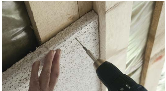
Positioning the screws or the acoustic panels with auxiliary lath. Make sure that there is enough space at the end of the panel to prevent the edge from displacing. Make sure the screw head is flush to the surface of the panel. The auxiliary lath is removed after installing the first row of panels. Screw pattern, see pages 5, 6 and 7.
