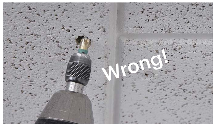
Not this way! – The screw head must be flush with the surface of the panel. A depth gauge should be used to prevent the over-driving of screws into the face of the panel.
