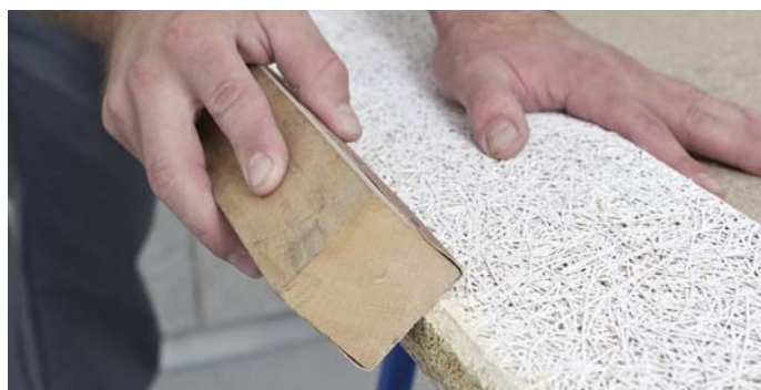
Creating the edge bevel – The bevel is formed with coarse sand paper, belt sander or a saw blade set on an angle.
