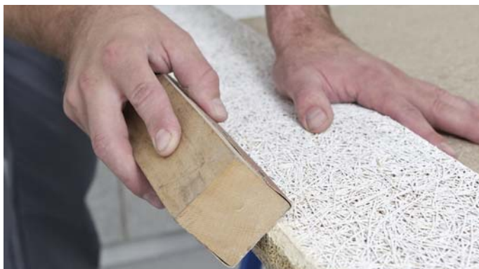
Creating the edge bevel – The bevel is formed with coarse sand paper, belt sander or a saw blade set on an angle.
