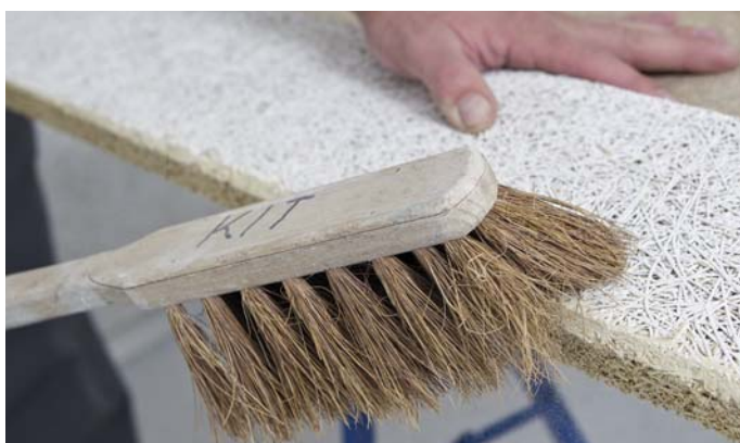
Remove any dust with a soft brush.
