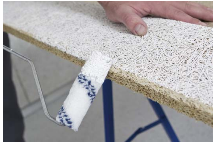
Painting the bevel – Use a brush or a thin paint roller to apply the paint.
